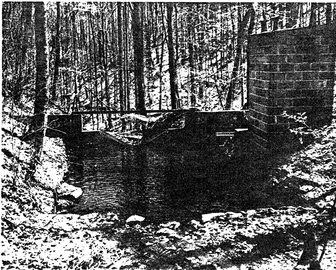
Weir, stilling basin, and gage house on a study watershed.
