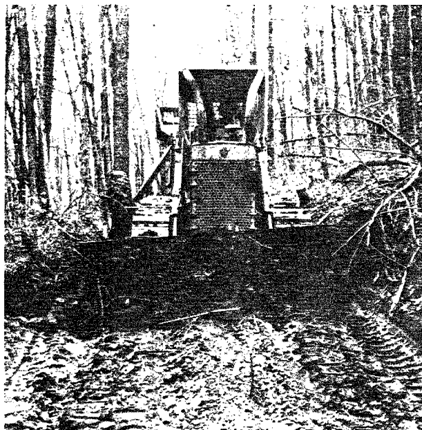
Bulldozing a water bar. Careful designing of skid roads was an important feature of watershed research on the Forest.
